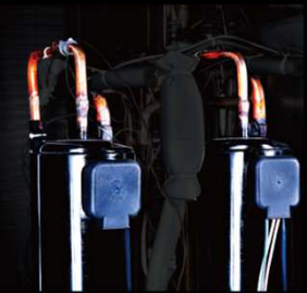
Multiple large-capacity all inverter compressors
